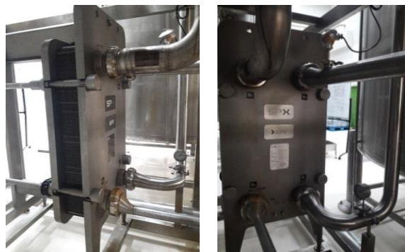
Gambar 1: Plate Heat Exchanger tipe Q030E RKS –10/1
